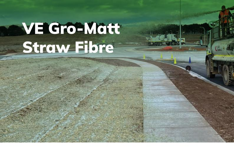
A hydraulically applied, one-step revegetation and soil binding solution, VE Gro-Matt Straw Fibre leads to improved soil health and self sustaining vegetation.
